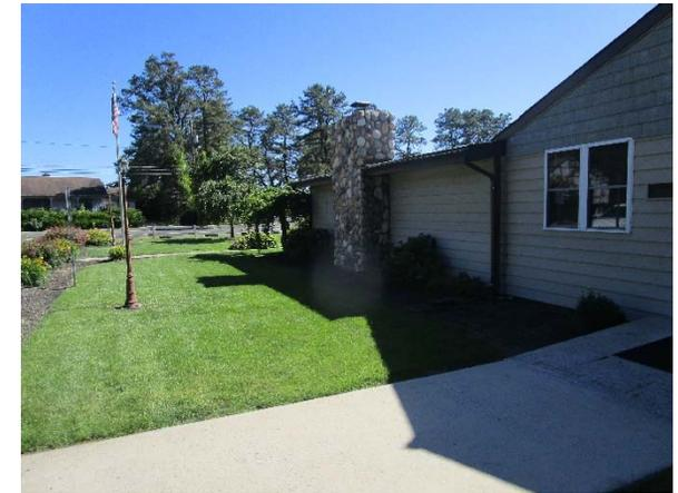
A rain garden can be installed at the east side of the building closest to the handicap parking spaces to allow stormwater runoff from the roof to infiltrate the ground and reduce the amount of runoff. A preliminary soil assessment suggests that the soils have suitable drainage characteristics for green infrastructure.
