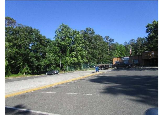
Parking spaces in front of the building can be converted into pervious pavement to allow the stormwater runoff from the road, roof, and parking lot to infiltrate the ground. The current conditions of the parking lot are poor; there are visible signs of erosion due to stormwater and cracking through the area. A preliminary soil assessment suggests that the soils have suitable drainage characteristics for green infrastructure.
